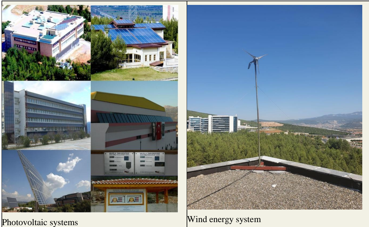
Figure 6: PV and Wind Energy Systems
