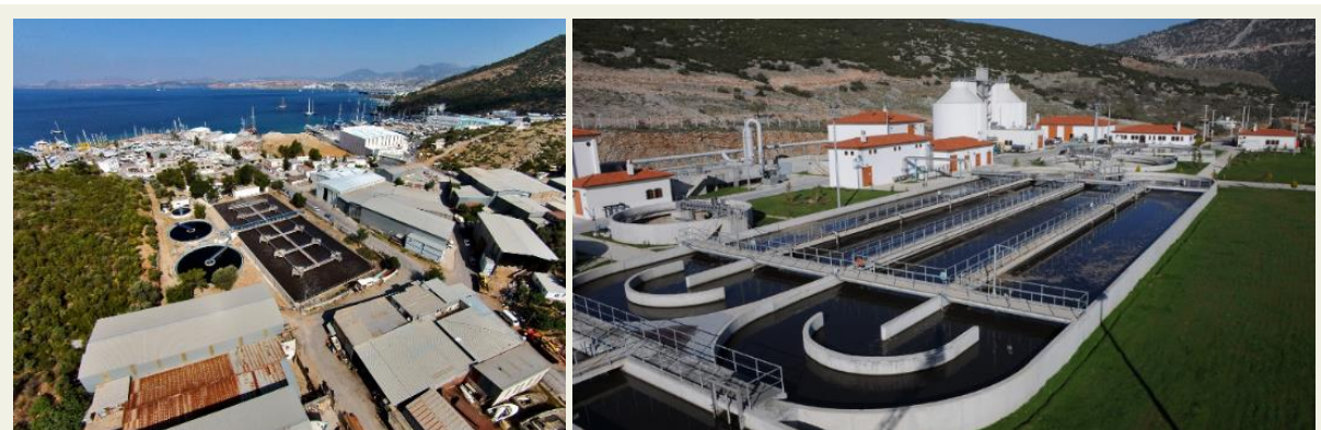
Figure 13: Muğla Conventional Wastewater Treatment Facility
