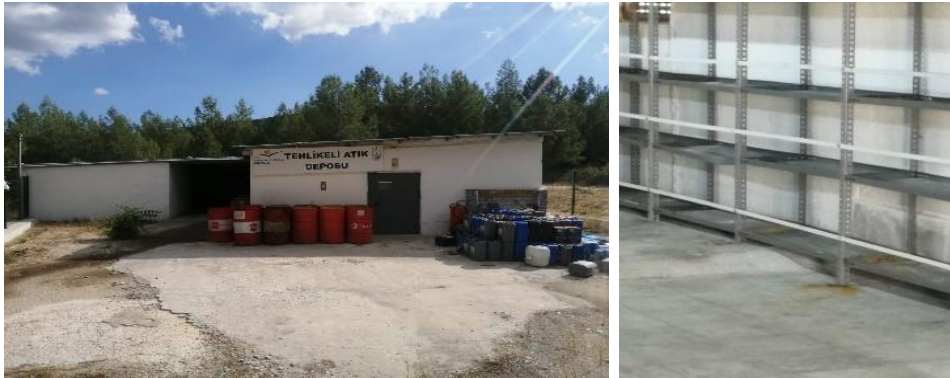
Figure 12: Hazardous Waste Warehouse
